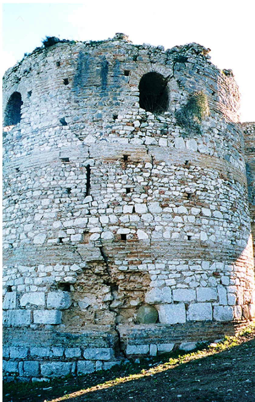
Fig. 33. Nikopolis. W part of the fortifications, tower. Type 1 masonry.
